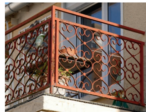
▶ Garde-corps sur balcon
